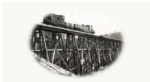
Stony Creek Trestle Bridge 4km west of Nowa Nowa
