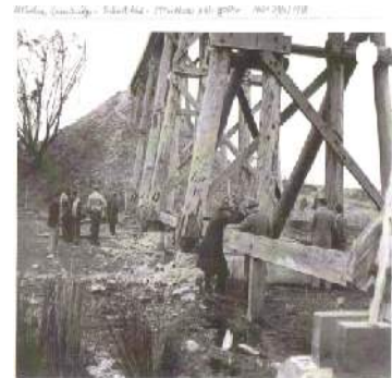
Officials looking at the damage
