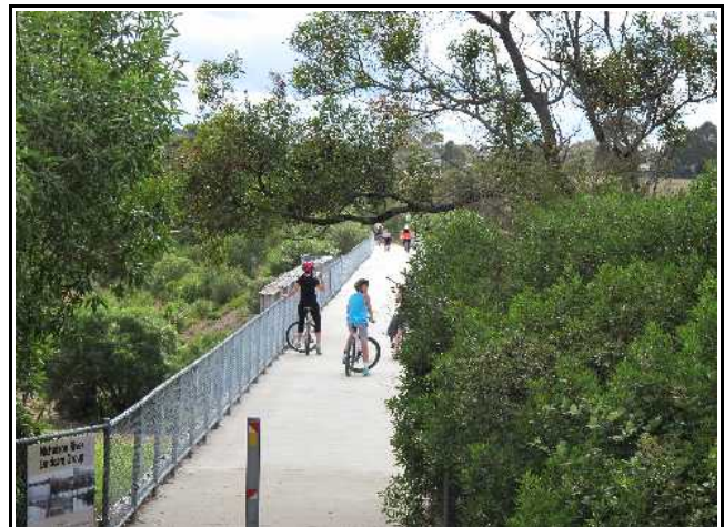
Nicholson River bridge.
