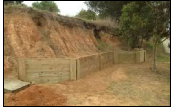
The new retaining wall work at Bairnsdale
