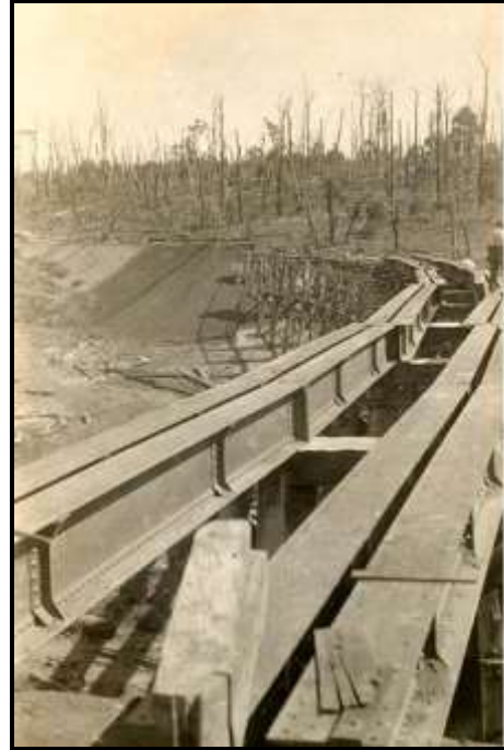
O'Grady's Bridge under construction circa 1914
