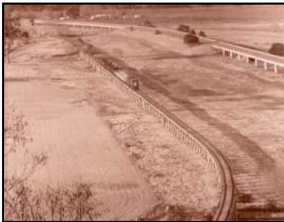
A view from Grandview – the last train crossing the Orbost flats on the viaduct
