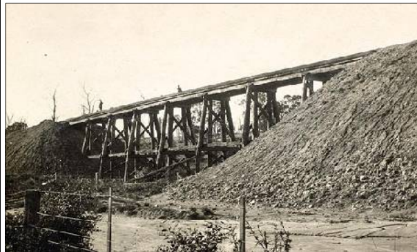
The bridge a little later 1914-15.
