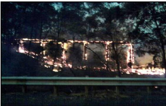
The bridge alight on the night of February 1 2011.
