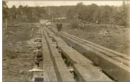
1914-15. Timbers have been laid across the piers but are not yet fastened in place.
